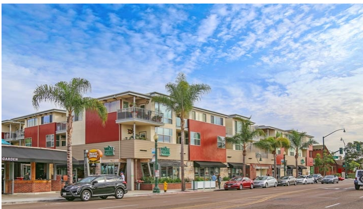
Figure 12: Pacific Station Development, Encinitas
