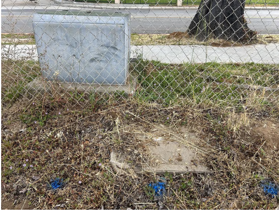
Photograph 13. Utility boxes near the northern corner along Horne Street.
